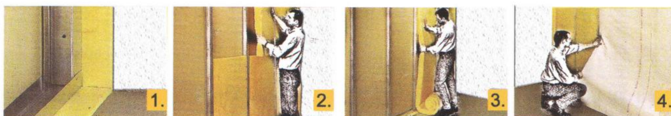
Process for installing Glass wool insulation in the walls of a building built
